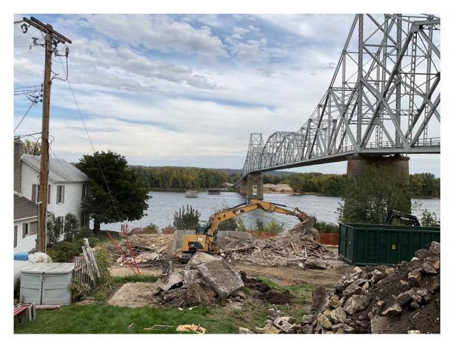
Known originally as the Black Hawk Bridge, the structure has a narrow deck at only 21 ft., with no shoulders. This makes it problematic for drivers with mechanical issues to pull over safely. The new bridge will be wider, at 40 ft. (two 12-ft. driving lanes with 8-ft. shoulders on both sides).
